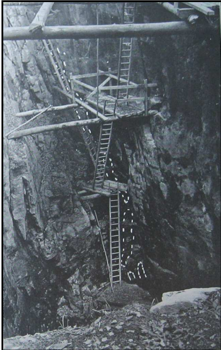
South Eastern part of the Frankengruvan open-cut; the uranium-bearing zone was marked with white paint behind the ladders (Photos from the following publication: Geol. Fören. Förhandl., v83, 129-143 (1961))
