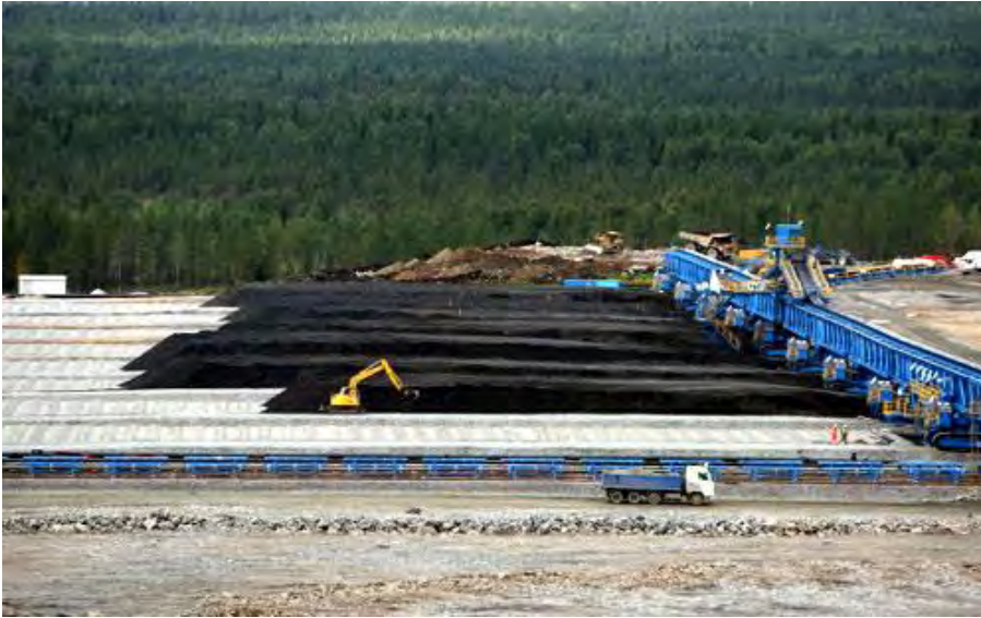
Talvivaara Project, Finland
